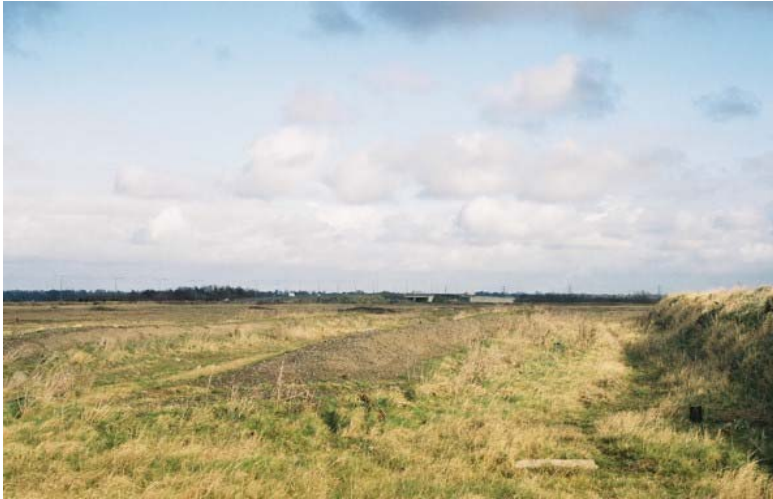
Sand capping to block source-receptor pathway.
